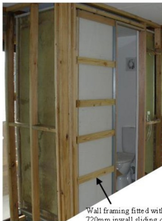
Brace screwed to bathroom flange
