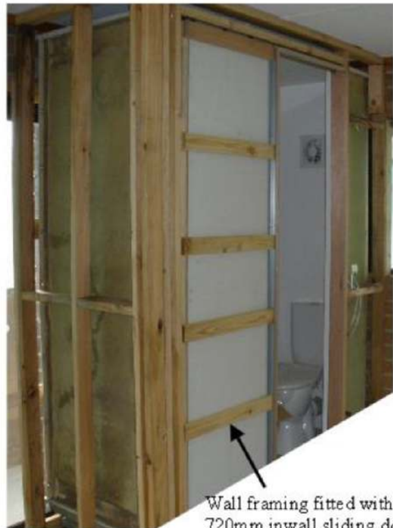
Brace screwed to bathroom flange
