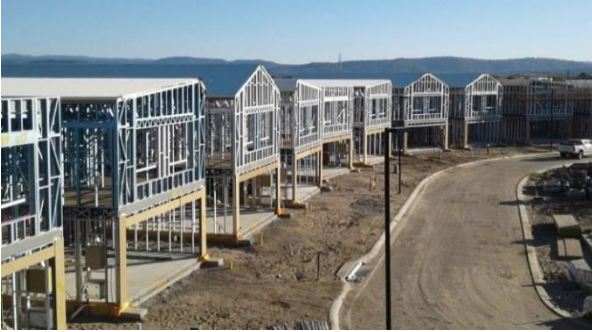
Pre-fab Steel Frame – Duplex House
