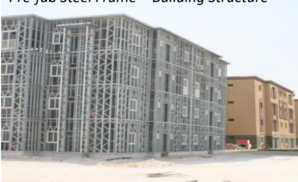
Pre-fab Steel Frame – Building Structure
