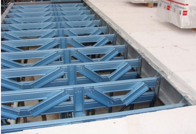
Pre-fab Steel Frame – Upper Floor
